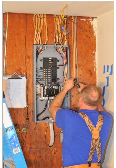
A contractor replacing a panel.
